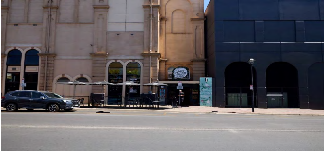
11. Norwood Town Hall Complex 49 George Street, Norwood
