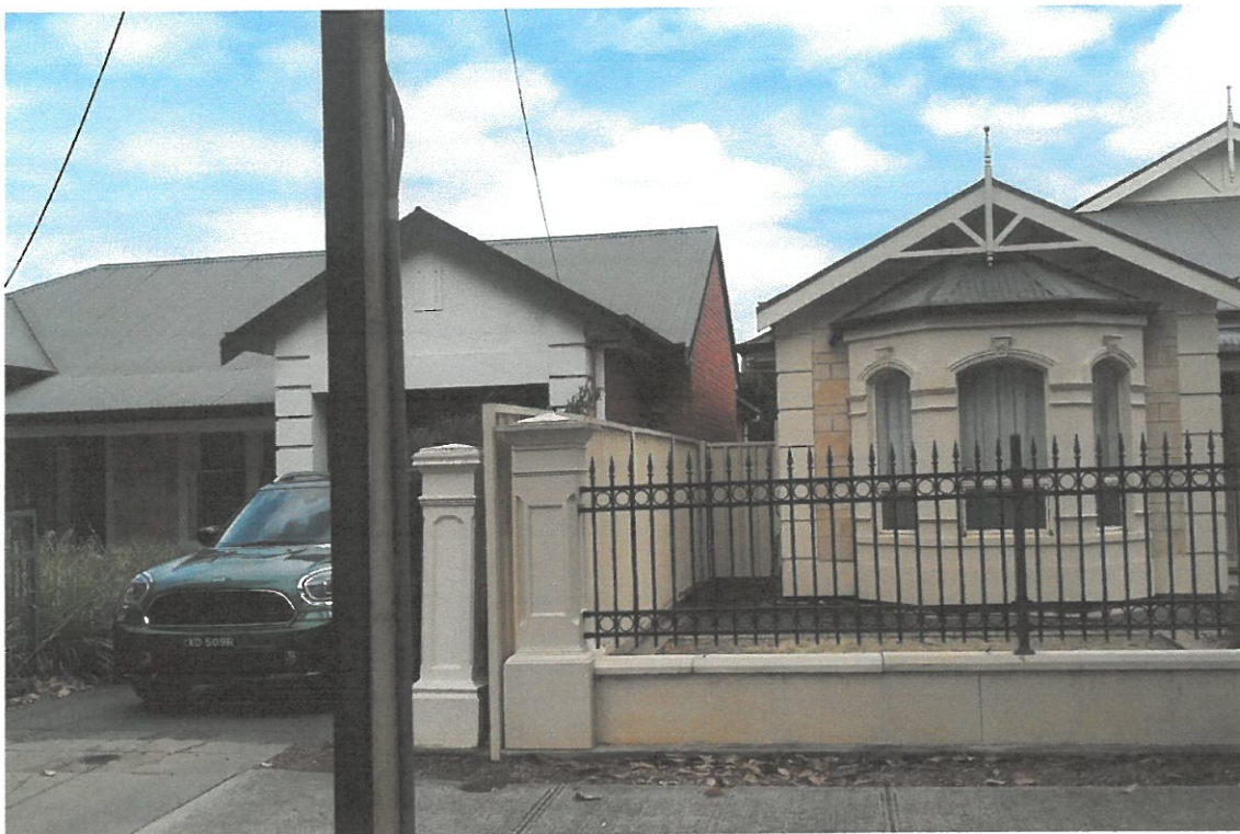
78 EIGHTH AVENUE (EXCESSIVE HEIGHTS + GABLE ENDS)
