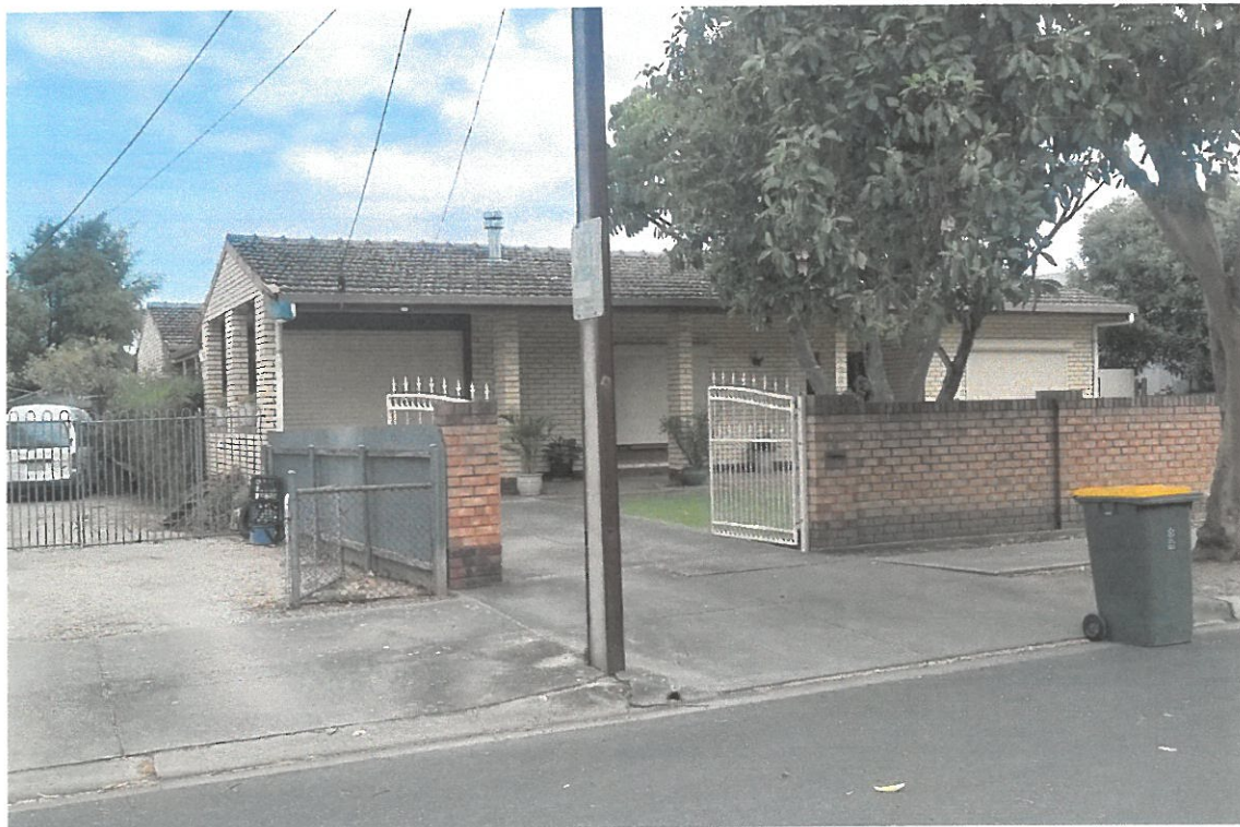
76 EIGHTH AVE. (2 SECTIONS OF HOKE ON BOUNDARY.) EXCESSIVE HEIGHT & CABLES.
