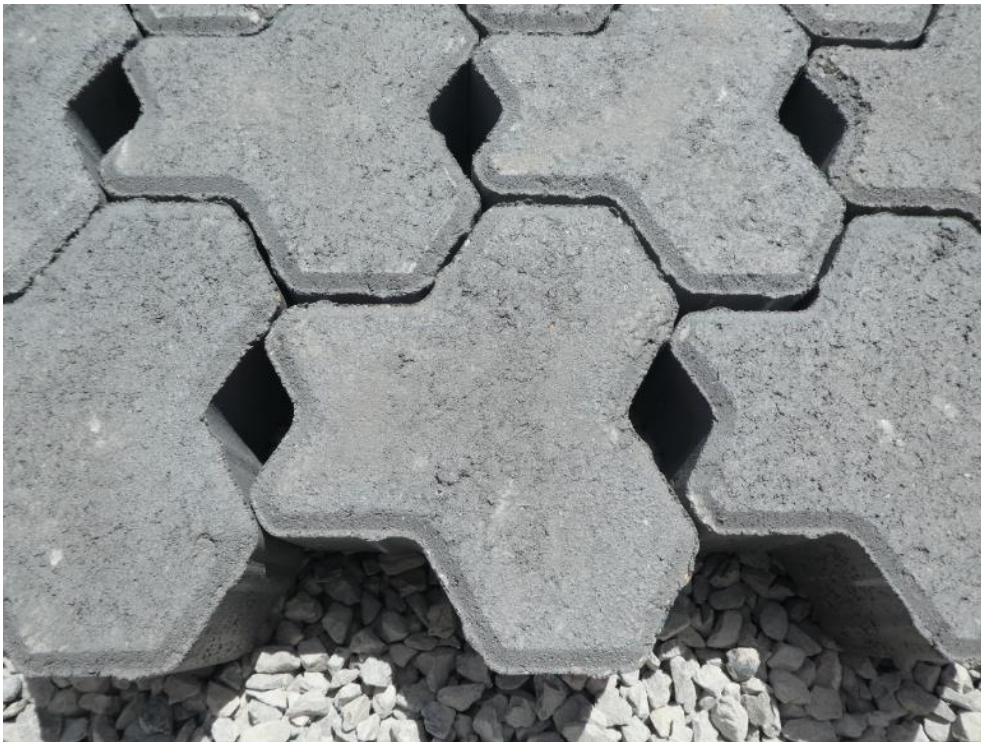
Figure 2: 'Ecotrihex' pavers on washed aggregate drainage layer.
