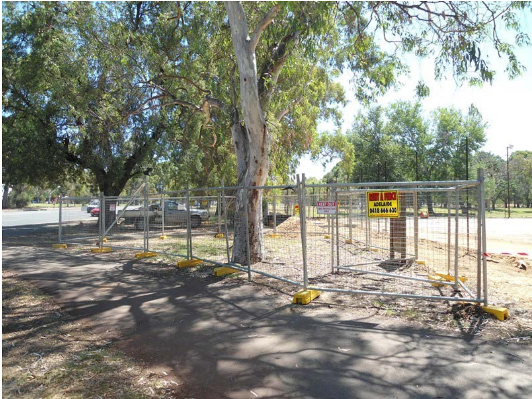
Figure 2: Typical TPZ fencing.
