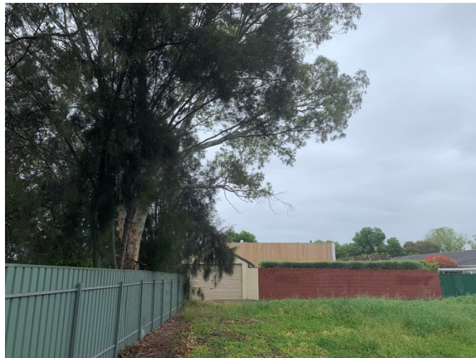
Photo 3: showing crown overhang.
