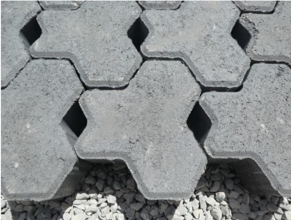
Figure 2: 'Ecotrihex' pavers on washed aggregate drainage layer.
