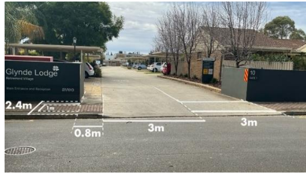
Photo 2: Eastern driveway crossover and fire hydrant
