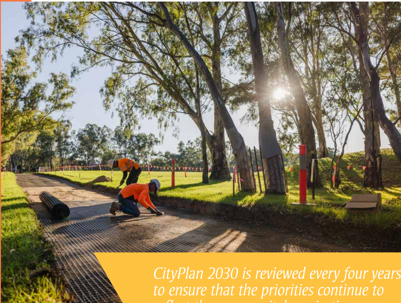
River Torrens Linear Park Shared Path
