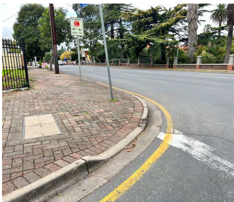
Figure 11 - Noncompliant Kerb Ramps
