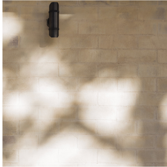
01 / BAGGED BRICK EXTERNAL WALLS
