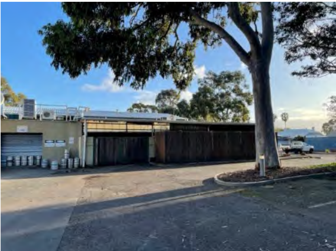
Figure 4: Rear Loading Dock and Service Area
