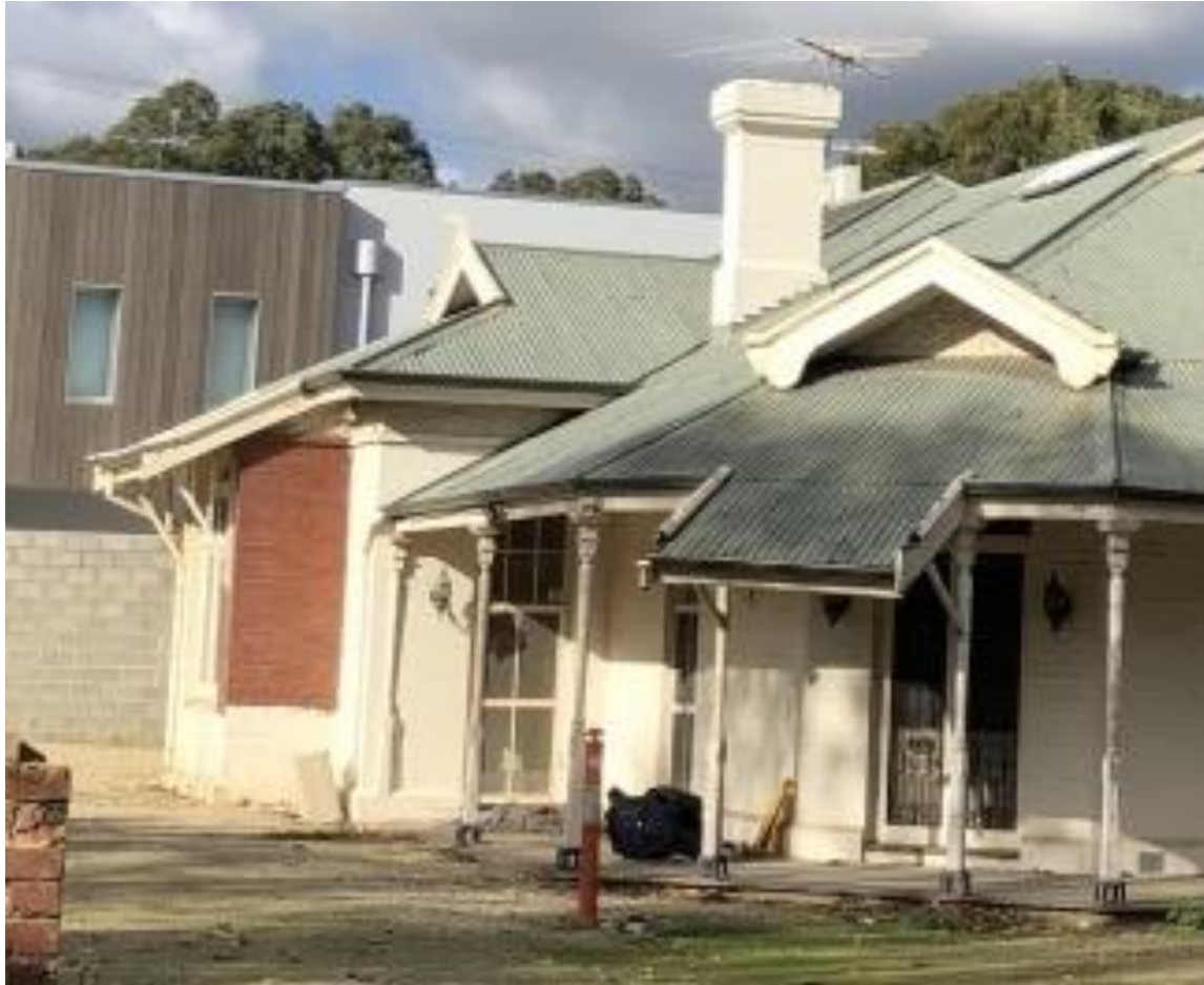
Original fine lined red brick finish sample section on bay window.
