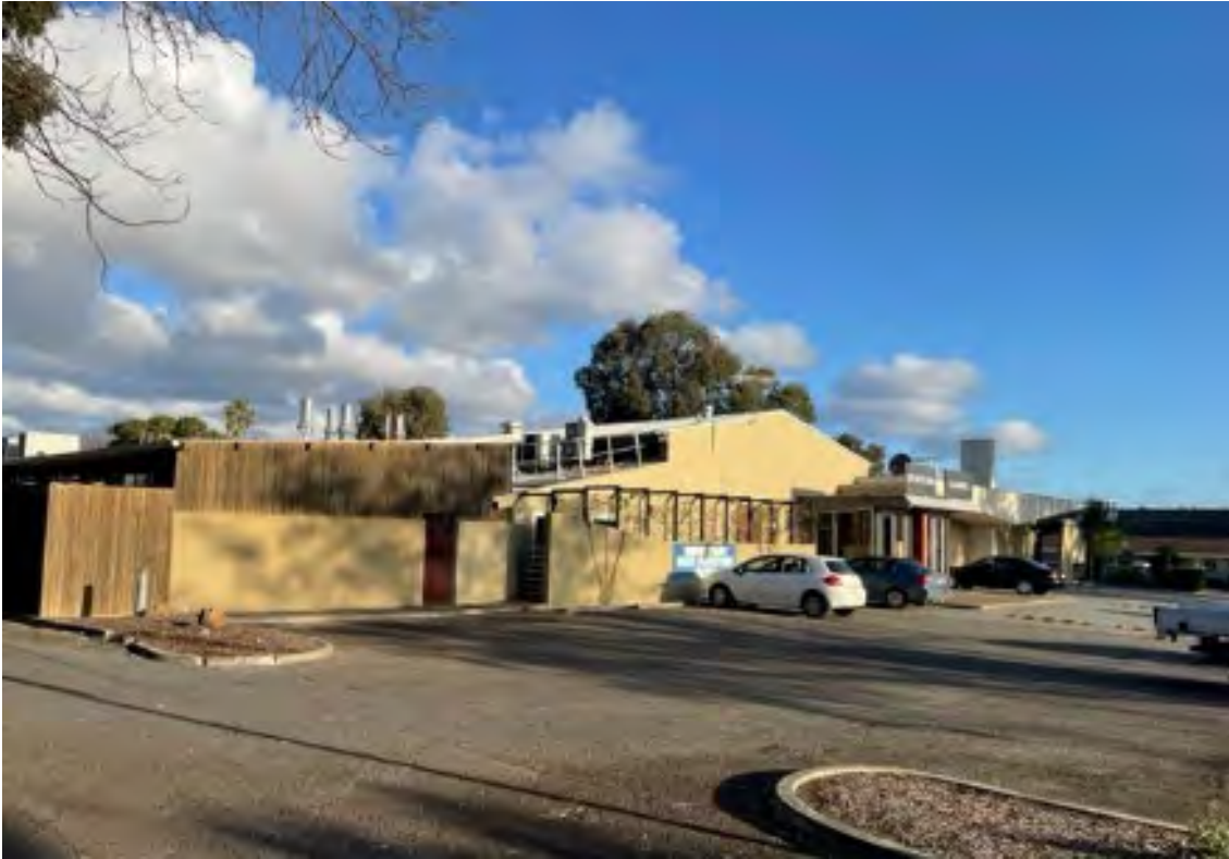
Figure 3: Rear Elevation of Building
